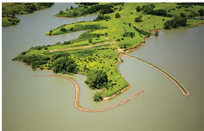
Construction of off-shore breakwaters and jetties, as shown above at Sherman Reservoir, are typically part of aquatic habitat improvements. In addition to providing improved fishing access, they create spawning shoals and feeding areas for game fish.
