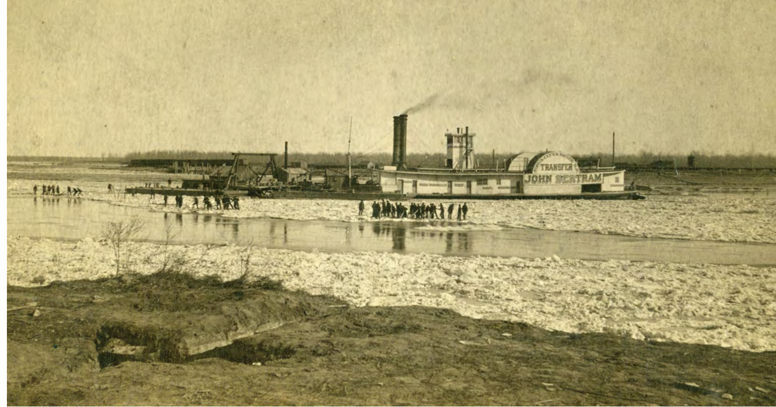
Travelers and workers often braved the icy Missouri River, just like these bridge workers near Rulo in 1886. History Nebraska RG2457-5-24
