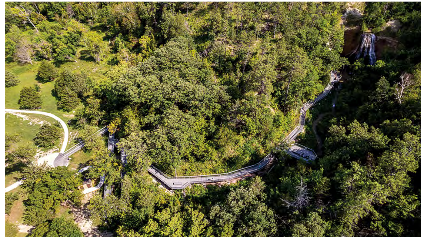
The new 500-foot walkway features wheelchair ramps, benches and a scenic vantage at its midpoint.
