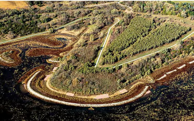
An Aquatic Habitat project at Cunningham Lake in Omaha included maintenance on a breakwater and resurfacing gravel spawning beds. ERIC FOWLER, NEBRASKALAND
