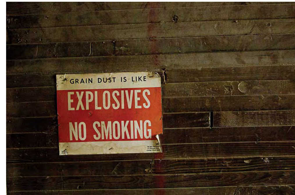
Tin-covered crib elevators were virtually indestructible and could have lasted decades. Their greatest threat was grain dust being ignited by a spark or careless smoker.
