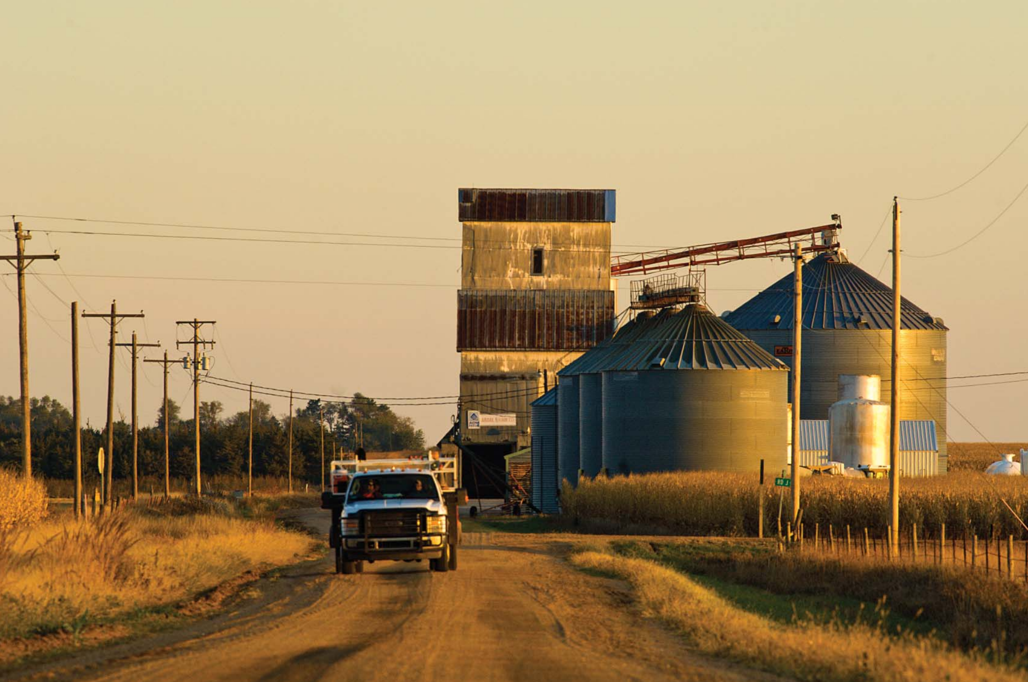
The little town of Abdal northwest of Superior was plotted in 1899, but before the town existed there was a crib elevator, serviced by the Kansas-Nebraska Railway Company. The original elevator could hold six railcars of grain. Today, a farming family owns it.
