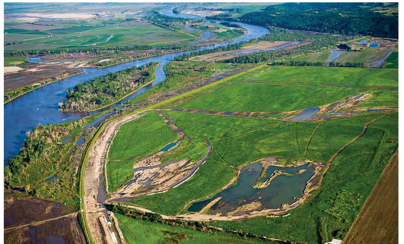
The Game and Parks Commission is allowing the U.S. Army Corps of Engineers to borrow soil from Peru Bottoms Wildlife Management Area to rebuild the levee along the area. The result will be wetlands that fill with groundwater when flows on the Missouri River are high, likely in the spring, as well as a diversity of plant life.
