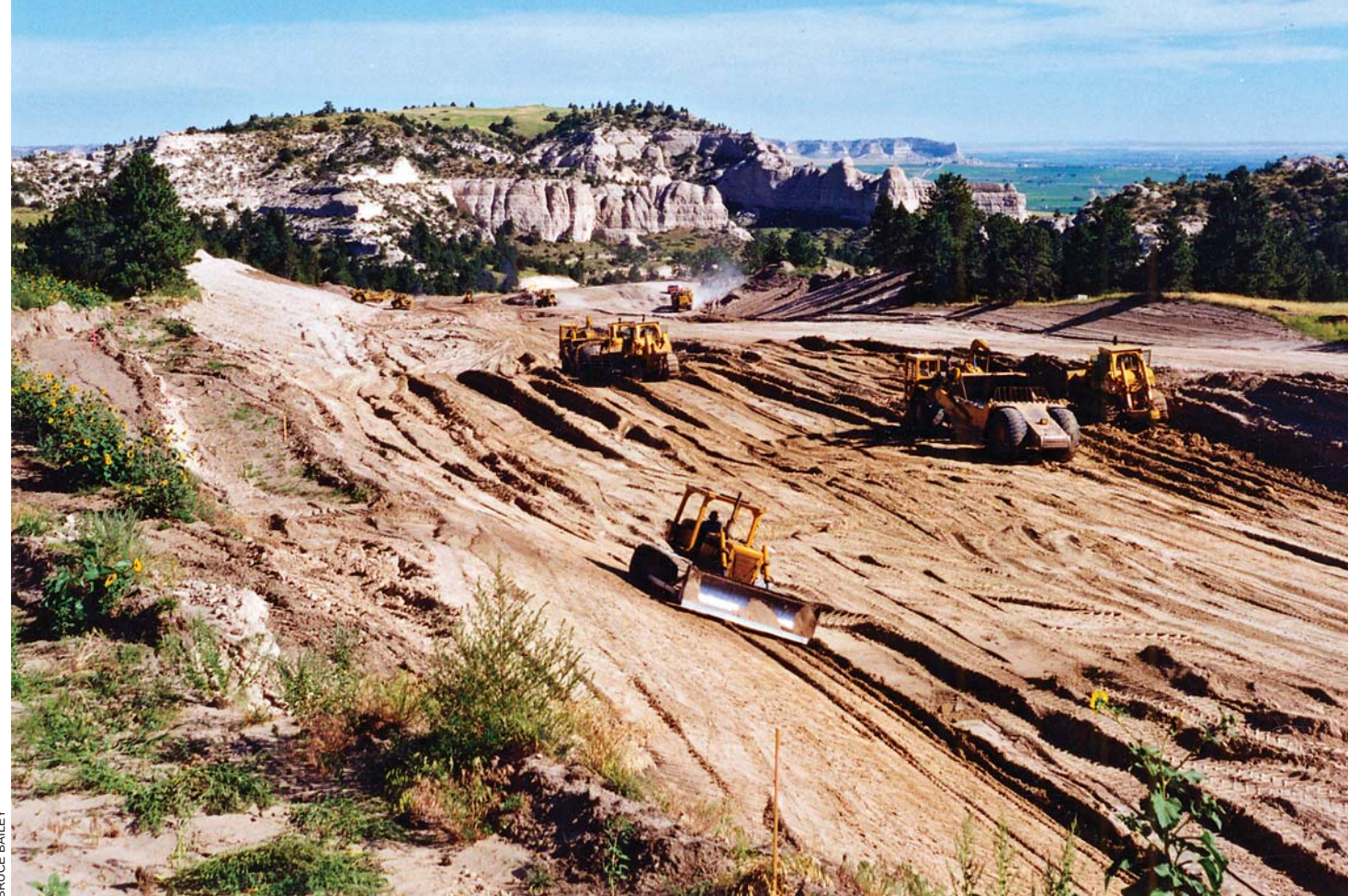
In 1999 bulldozers and scrapers remove the ancient river's upper channel deposits (foreground) at the Wildcat Grade during the widening of Nebraska Highway 71. In the background excavators are nearing the lower channel.
