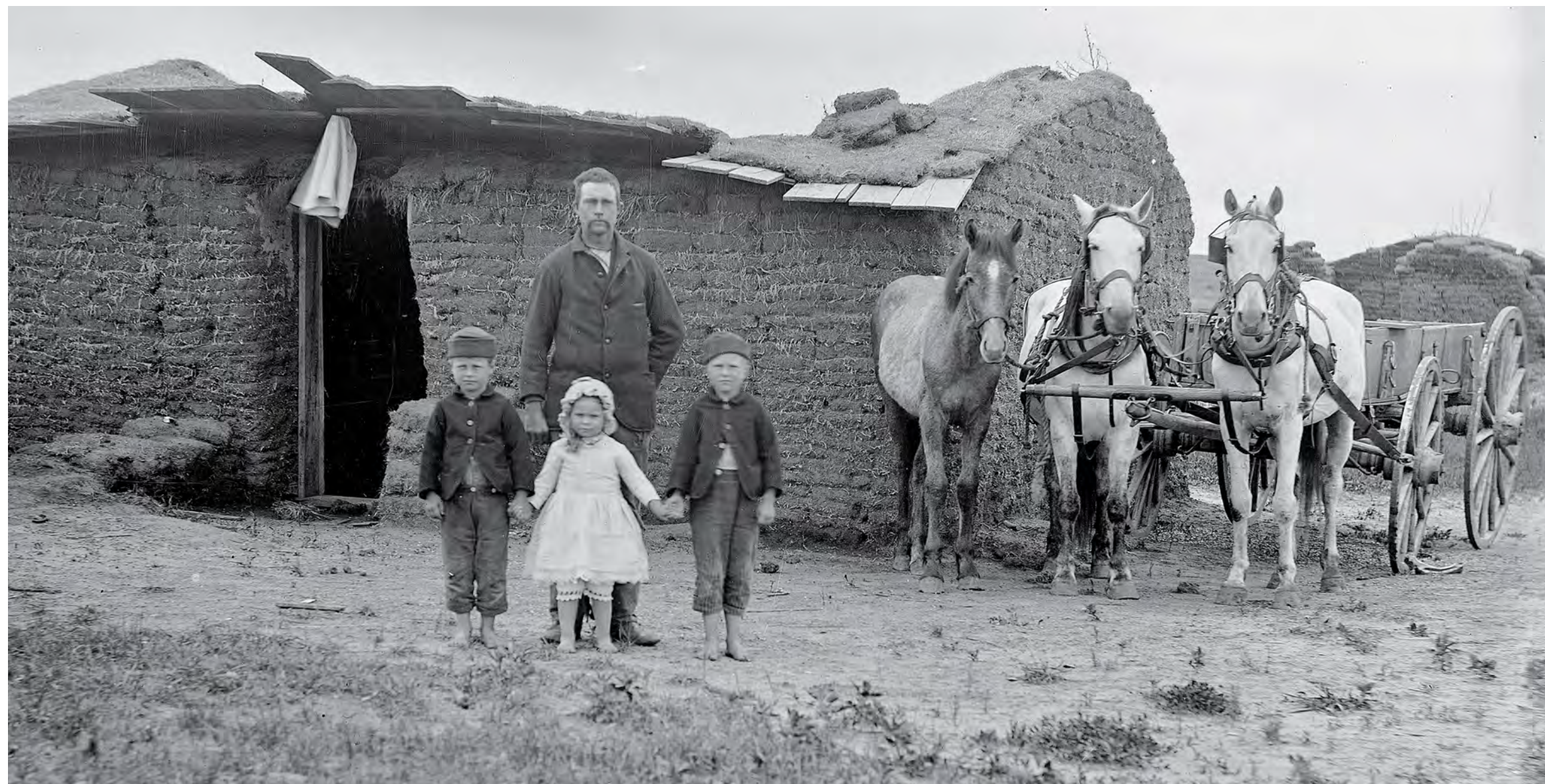
Heavy rains in 1887 caused Custer County widower George Barnes’s roof to collapse only 10 minutes after the family was out of bed. HISTORY NEBRASKA, RG2608-0-1190
