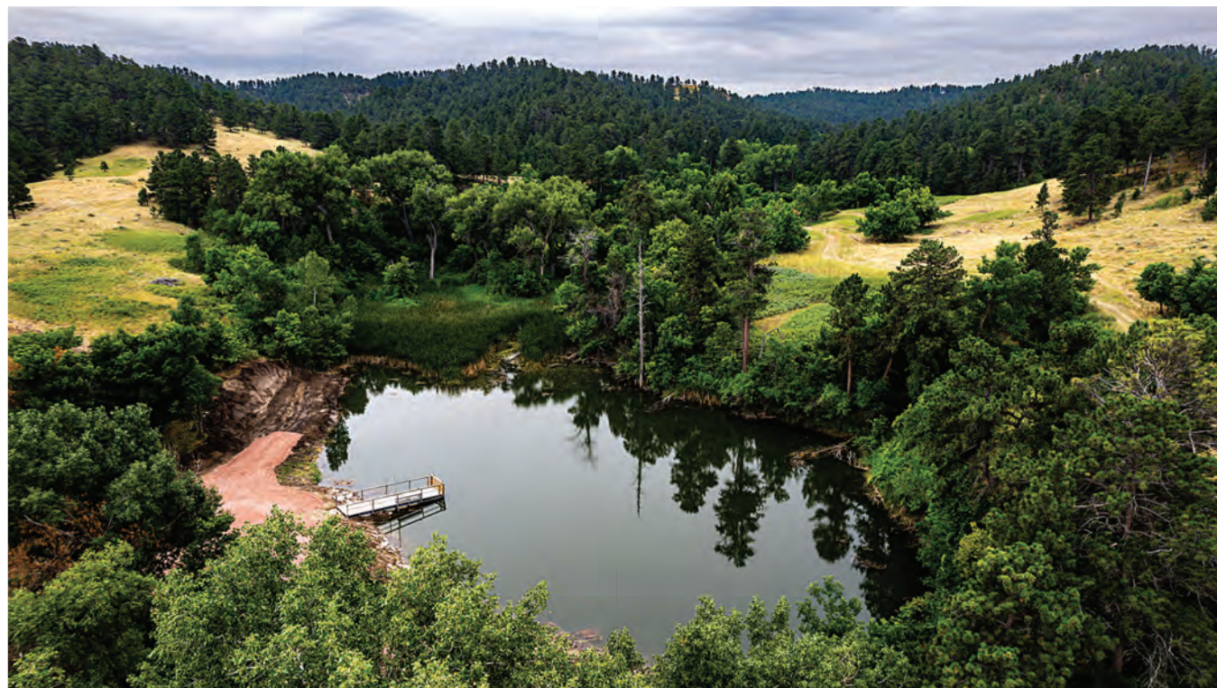
Shoreline clearing and grading and installation of a fishing dock improved access to the pond on East Monroe Creek at Gilbert Baker Wildlife Management Area north of Harrison. JUSTIN HAAG, NEBRASKALAND
