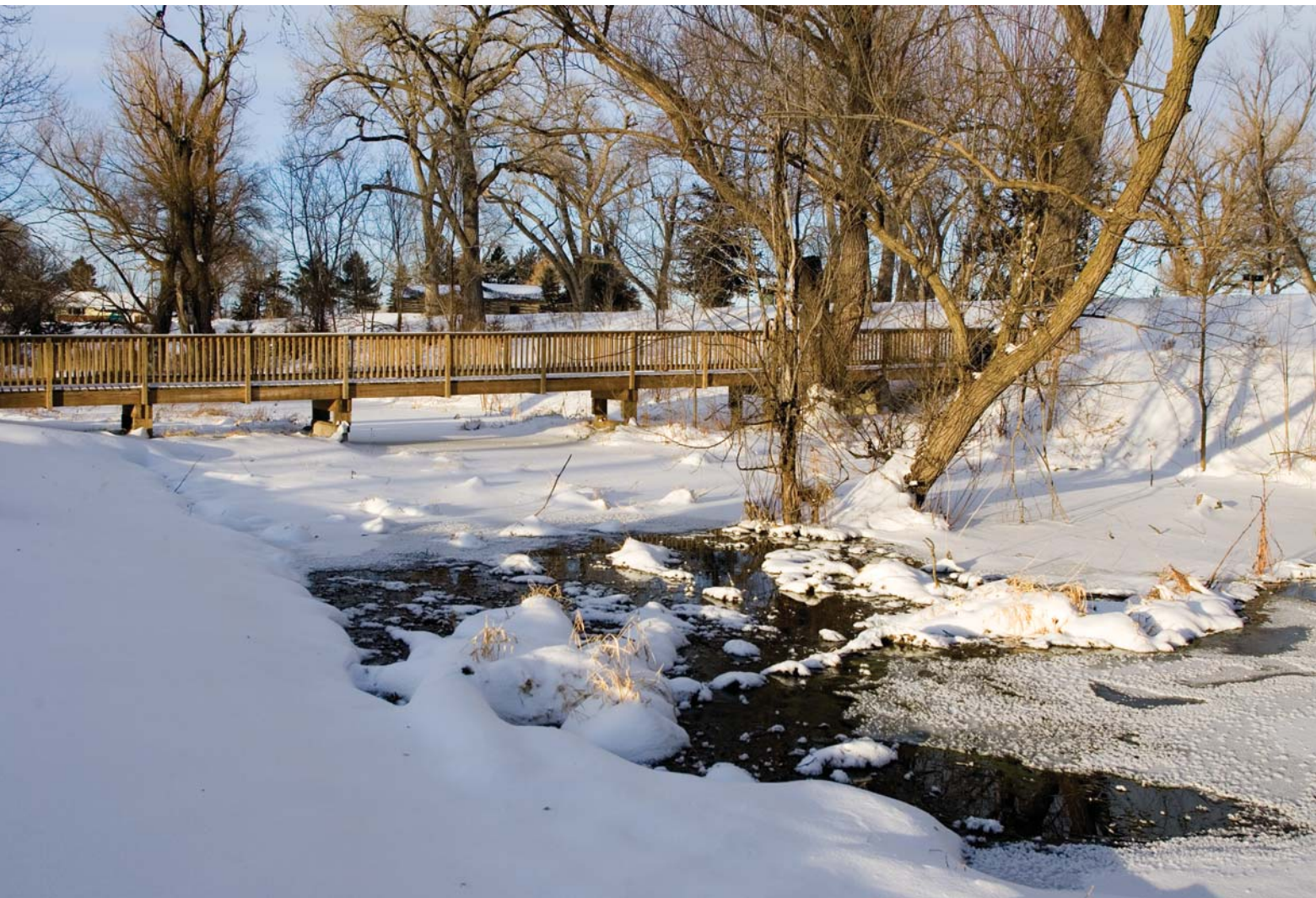
A new bridge constructed over Victoria Creek allows visitors foot access from their campsites to the oxbow lake.
