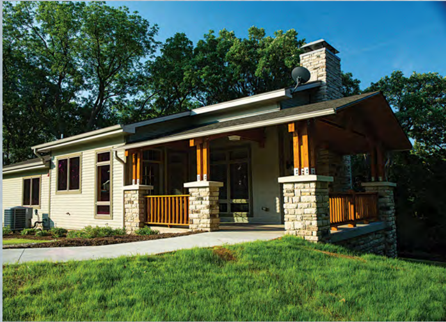
Funding from the Nebraska Game and Parks Foundation helped build this mini-lodge at Ponca State Park. JEFF KURRUS, NEBRASKALAND
