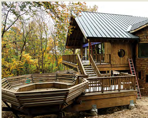
The nearly completed Treehouse Classroom at Schramm Park State Recreation Area.
