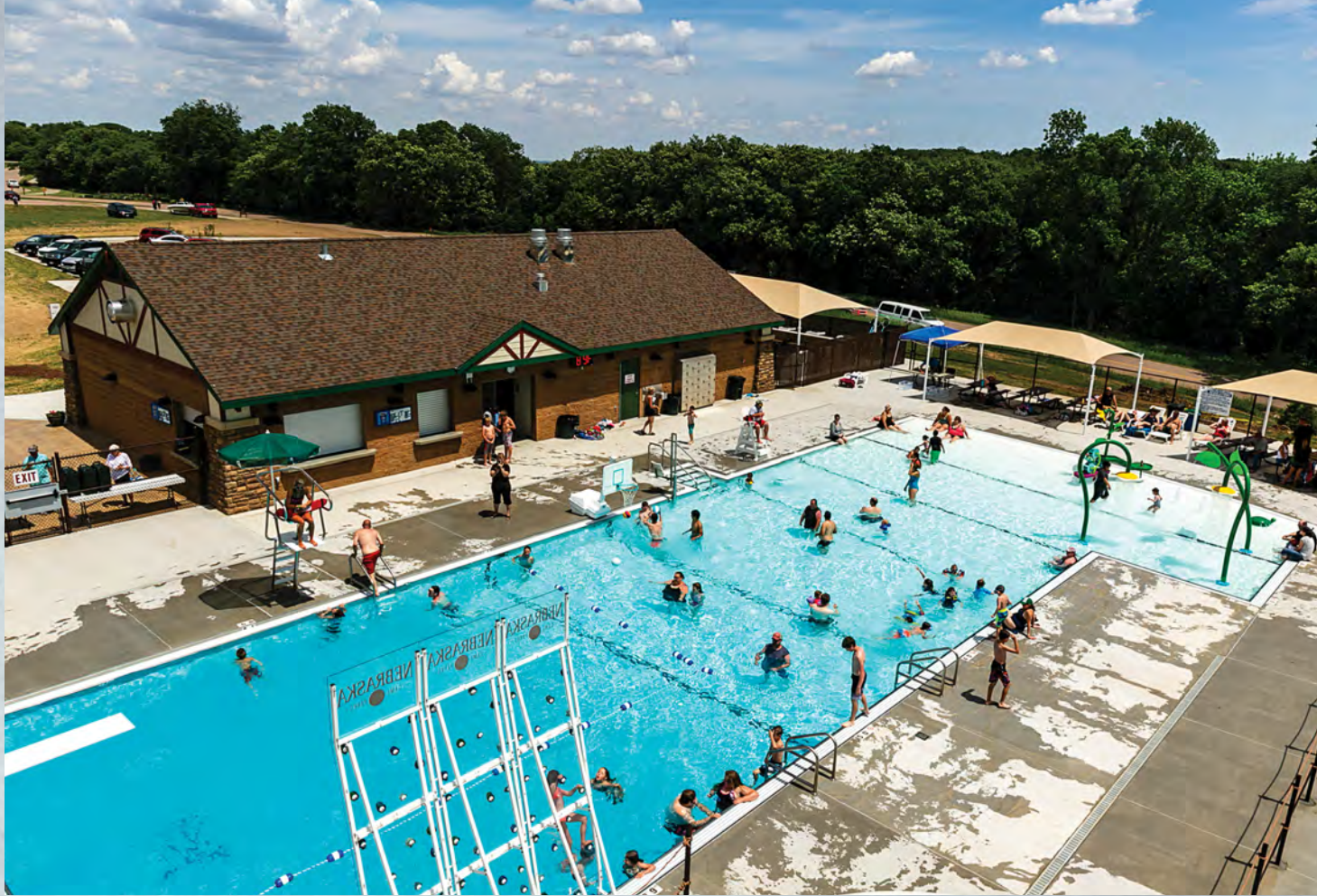
With Foundation assistance, Ponca State Park's aquatic center replaced a pool originally opened in 1956.
