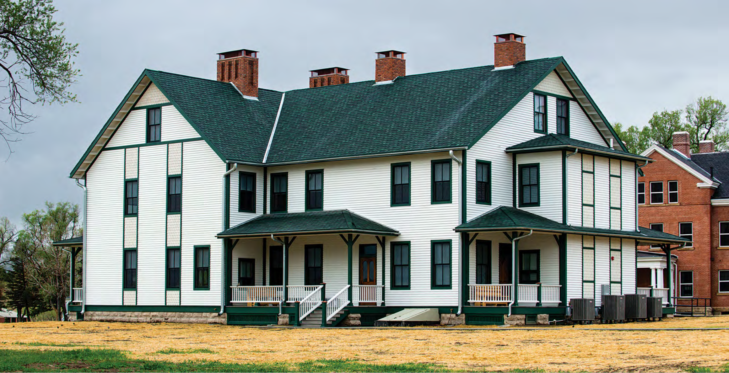
Since its completion in 2015, Fort Robinson State Park's 1891 Officers Quarters has become a destination for large groups looking for an authentic Western lodging experience. JUSTIN HAAG, NEBRASKALAND
