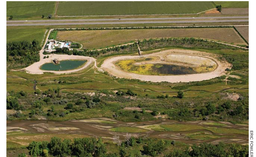
South of Interstate 80 near Wood River, the landowner violated the Federal Clean Water Act by using excavated material to form rings around these ponds. The excavated material is considered a pollutant and decreases Platte River water quality downstream. The landowner cooperated with clean up and was fined.
