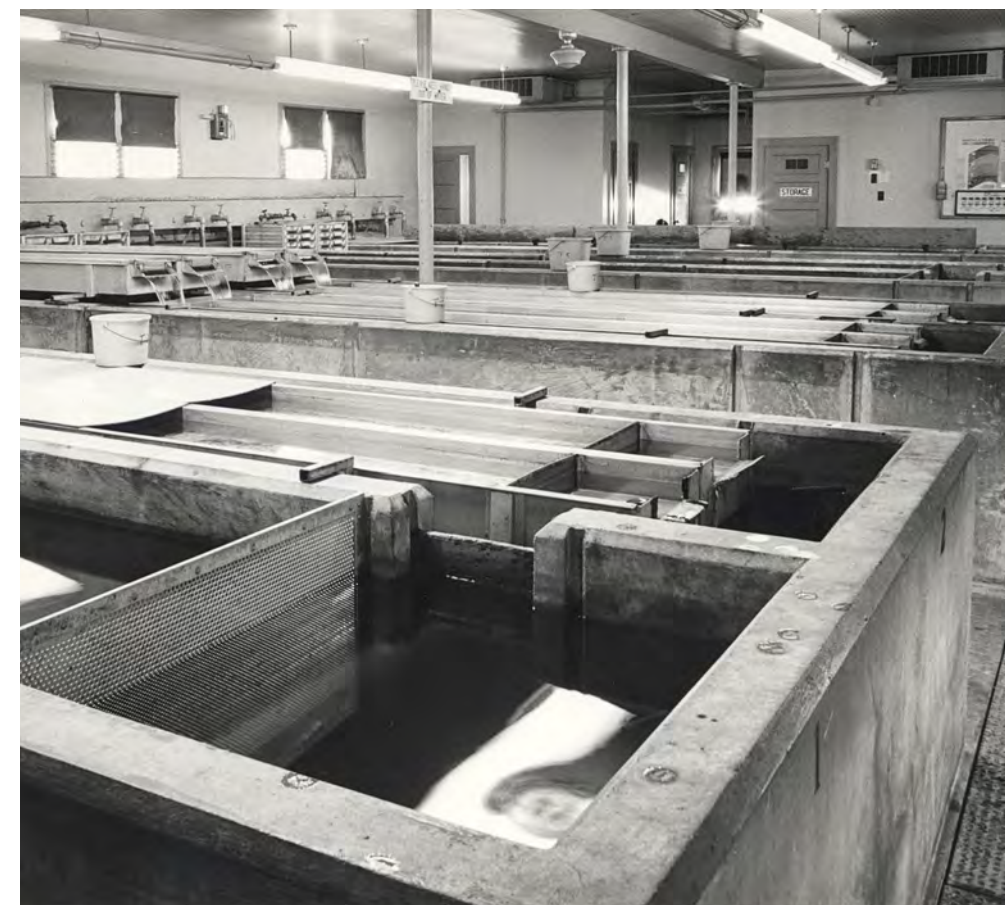
Interior of hatch house at the Crawford National Fish Hatchery in 1983. NGPC LIBRARY
