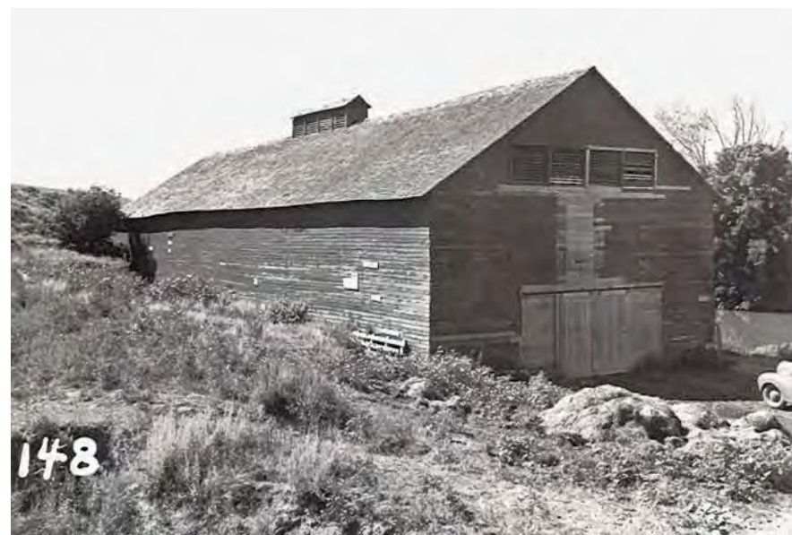
Constructed in 1904, the ice house at Fort Robinson served a vital role prior to artificial refrigeration. HISTORY NEBRASKA
