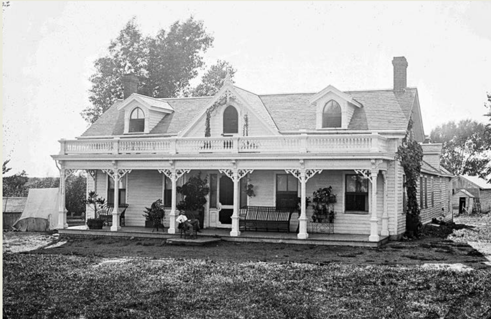
In 1875, the Mortons began calling their home “Arbor Lodge.” NSHS, RG2993-414
