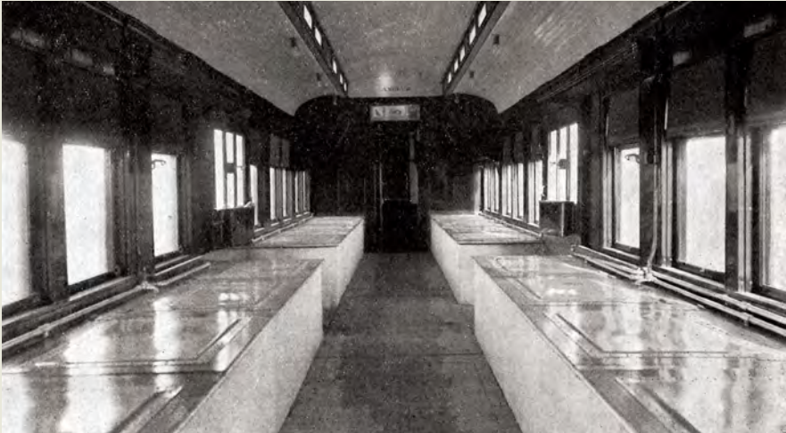
Interior view of the above photo fish car, the Angler, showing the tanks. Circa 1918. NGPC LIBRARY
