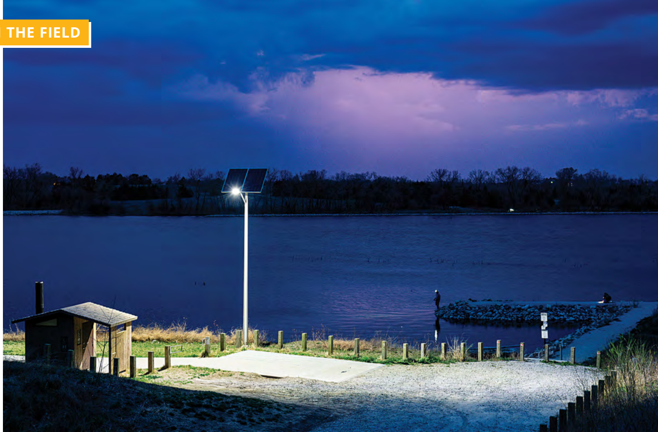
A solar light illuminates a brick house and parking area on the south side of Conestoga State Recreation Area near Denton in Lancaster County. ERIC FOWLER, NEBRASKALAND
