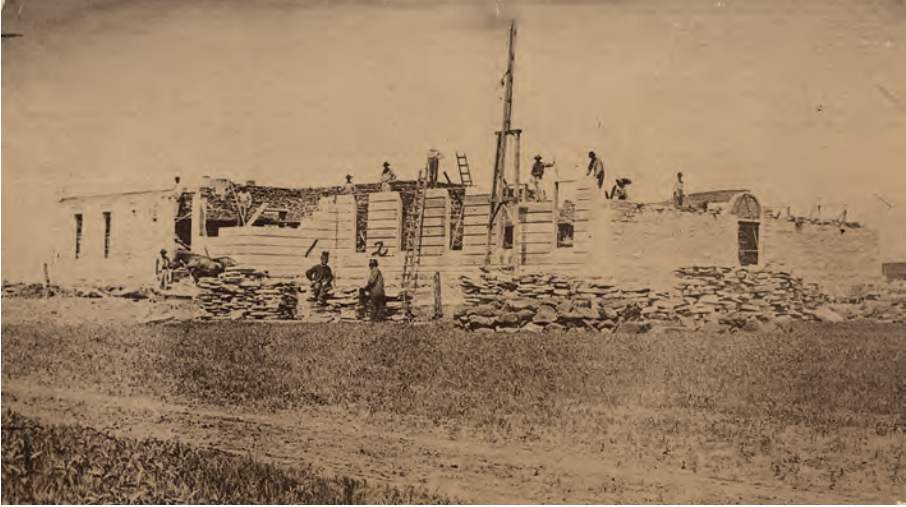
The new state capitol, shown here under construction in 1868, was a rush job to ensure that the legislature had a place to meet. Replaced in 1879-88, it stood on the site of the present capitol. NSHS RG1234-PH4-4
