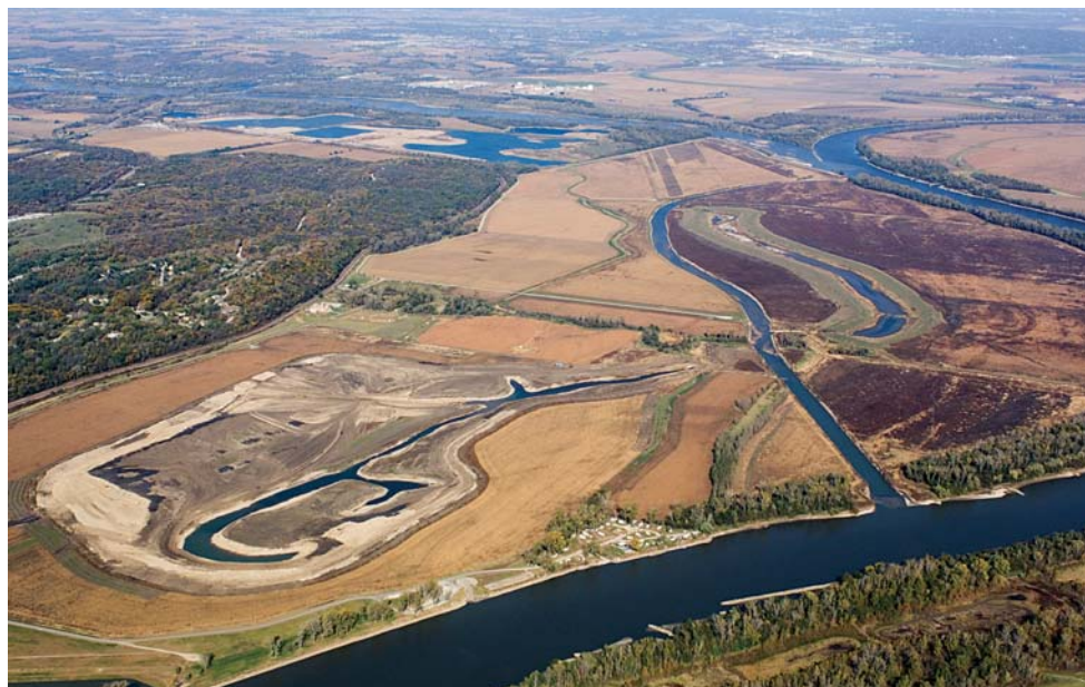
A recently completed flow-through chute at Schilling Wildlife Management Area near Plattsmouth has greatly increased fish and wildlife diversity in the area.
