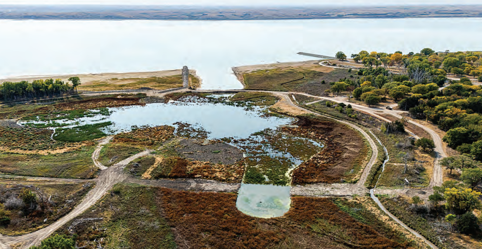
Water fills the portions of Methodist Cove where a channel was dug to connect the cove to the lake and sediment was removed as part of an aquatic ecosystem restoration project at Harlan County Lake. Soon after this photo was captured last fall, the construction road crossing the channel was removed. ERIC FOWLER, NEBRASKALAND
