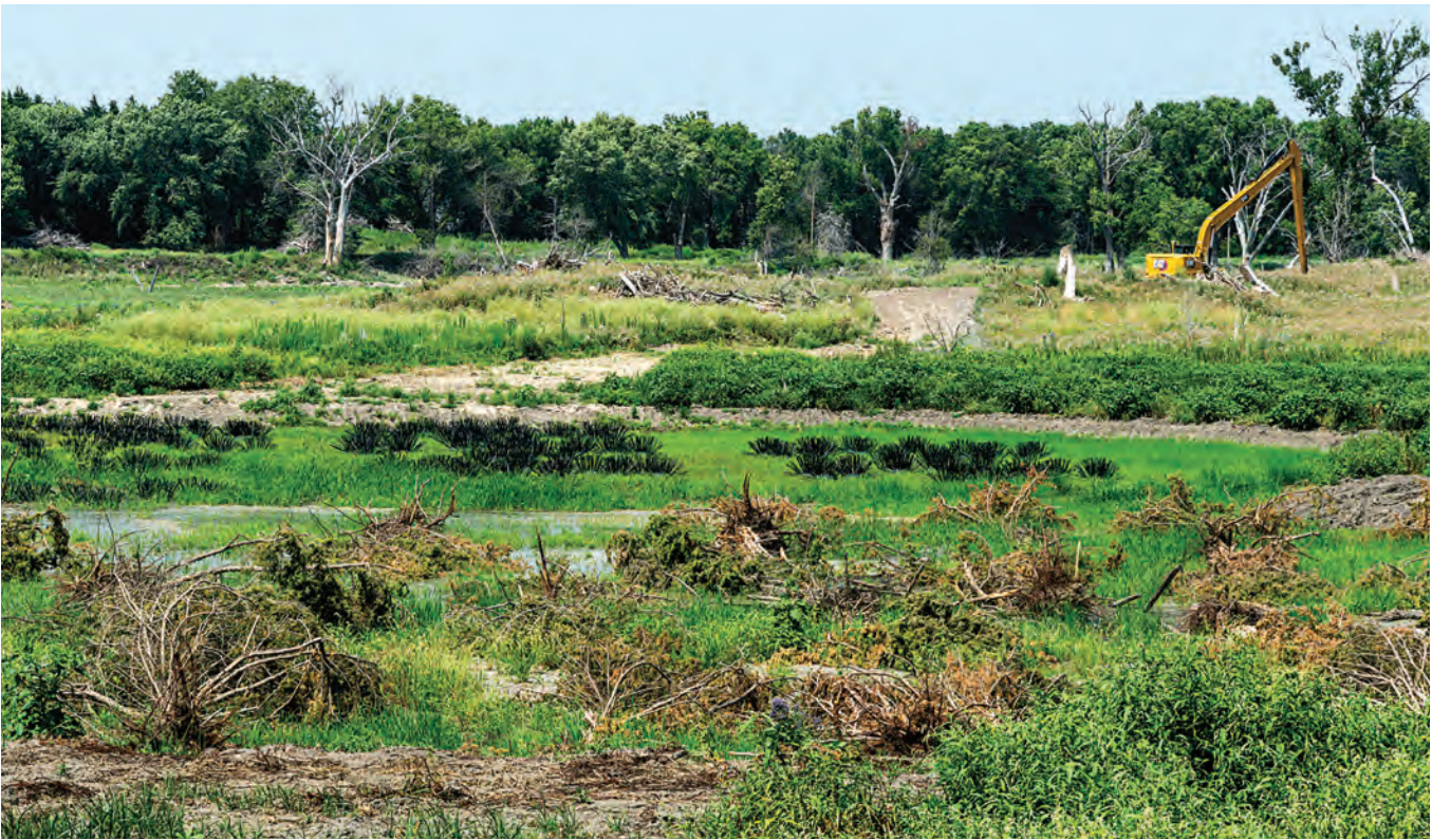
Artificial structures and cut cedar trees will serve as fish habitat in the area where sediment was excavated from Methodist Cove at Harlan County Lake. ERIC FOWLER, NEBRASKALAND
