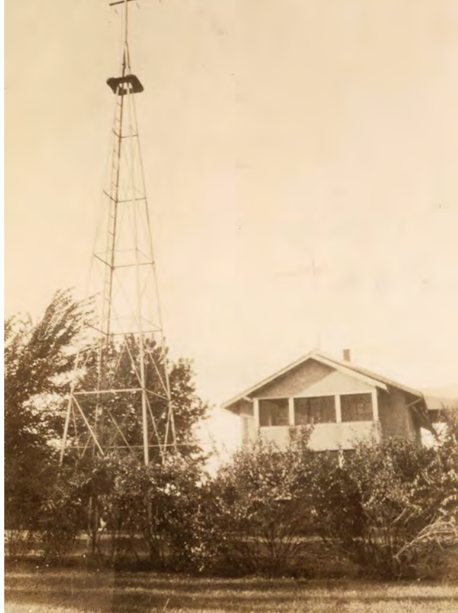
The KCGH tower at the hospital in Wayne. HISTORY NEBRASKA, RG3006.AM
