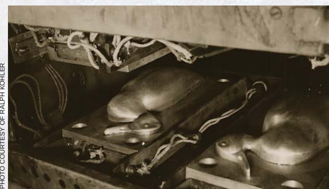
Ralph Kohler, one of the co-founders of K&W decoys, was a tool and die maker and owned a machine shop in Tekamah. He made the aluminum stamping dies for all the decoy models. A resin-impregnated forming board was shaped between the male and female dies under 200 tons of pressure.
