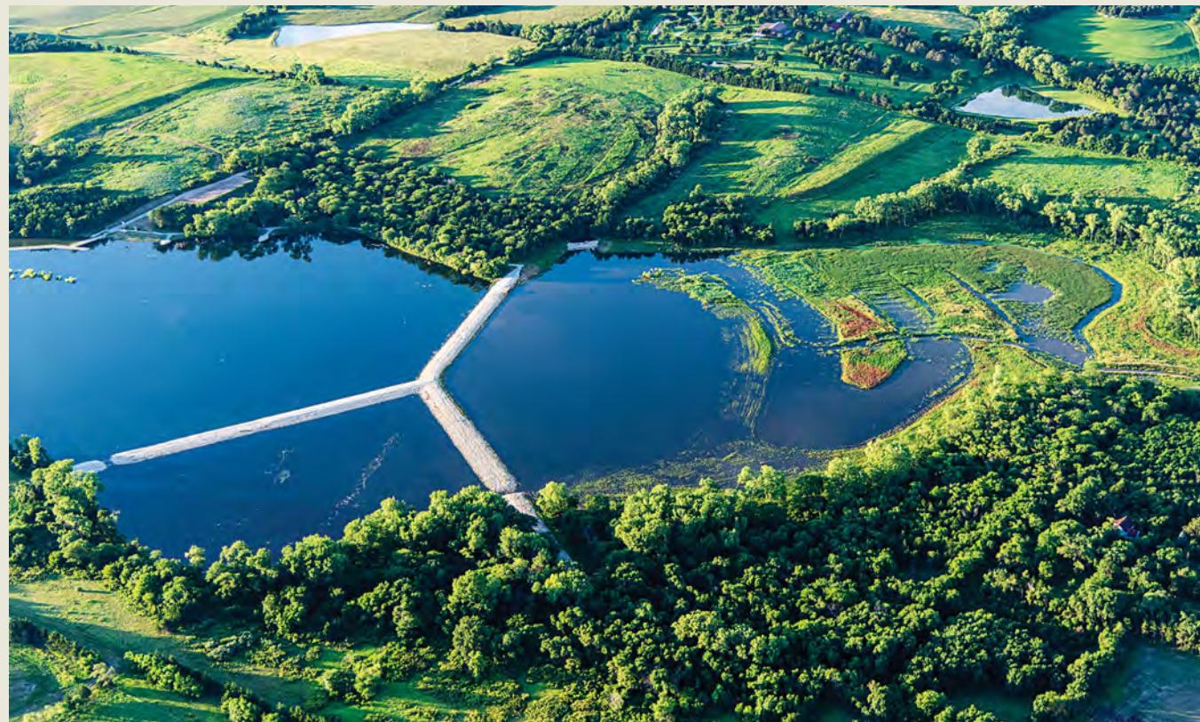
A three stage sediment trap in the upper end of the reservoir will keep silt out of the lake and maintain water quality, and also created wetland habitat for ducks, geese and shorebirds.
