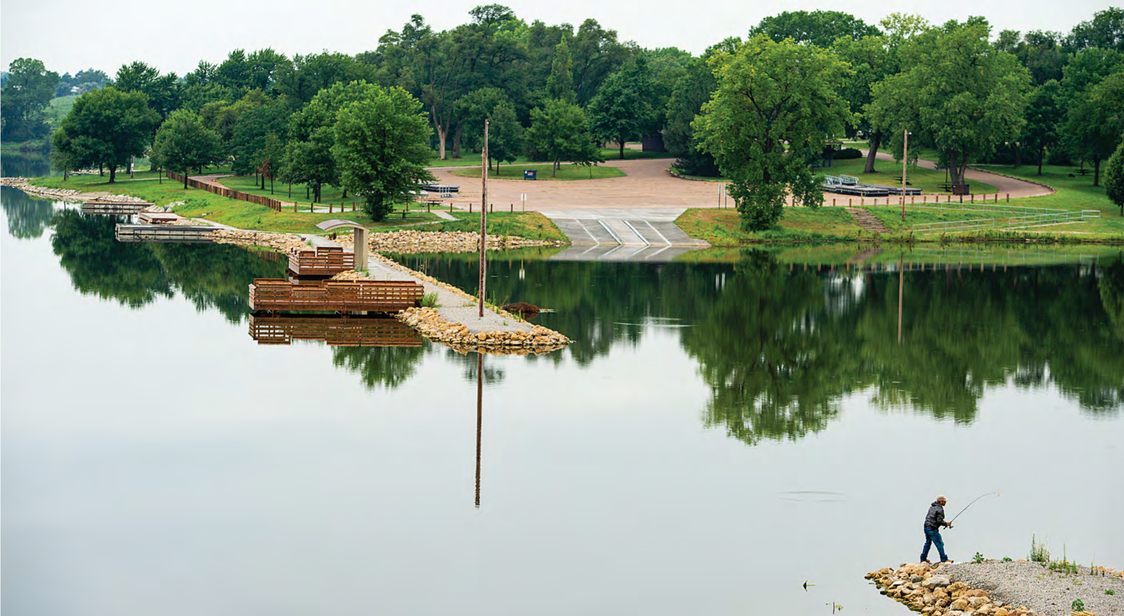
An angler fishes from one of the new breakwaters built to protect a bay and a new boat ramp in the northeastern corner of Conestoga Lake. Two fishing decks are found on the opposite breakwater.
