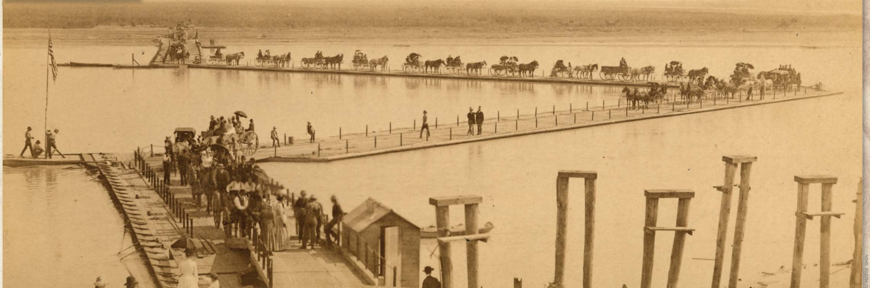
A pontoon bridge (also known as a floating bridge) that crossed the Missouri River near Nebraska City. The V-shaped portion could swing open for boats or flowing ice.
