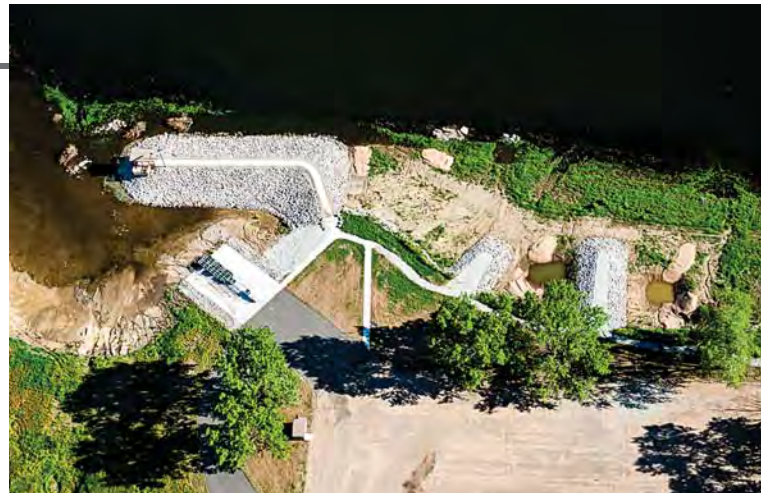
A new boat ramp, breakwaters, and numerous rock and tree pile and gravel beds built for fish habitat are visible in an aerial photo taken of Burchard Lake WMA before it refilled.
