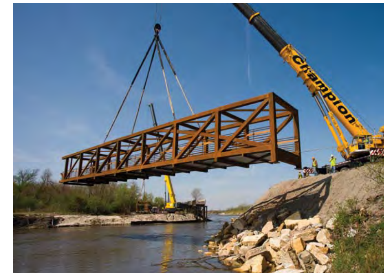
Tyson Construction crews swing the first of two segments of bridge into place over the Elkhorn River on the Cowboy Trail west of Norfolk.
