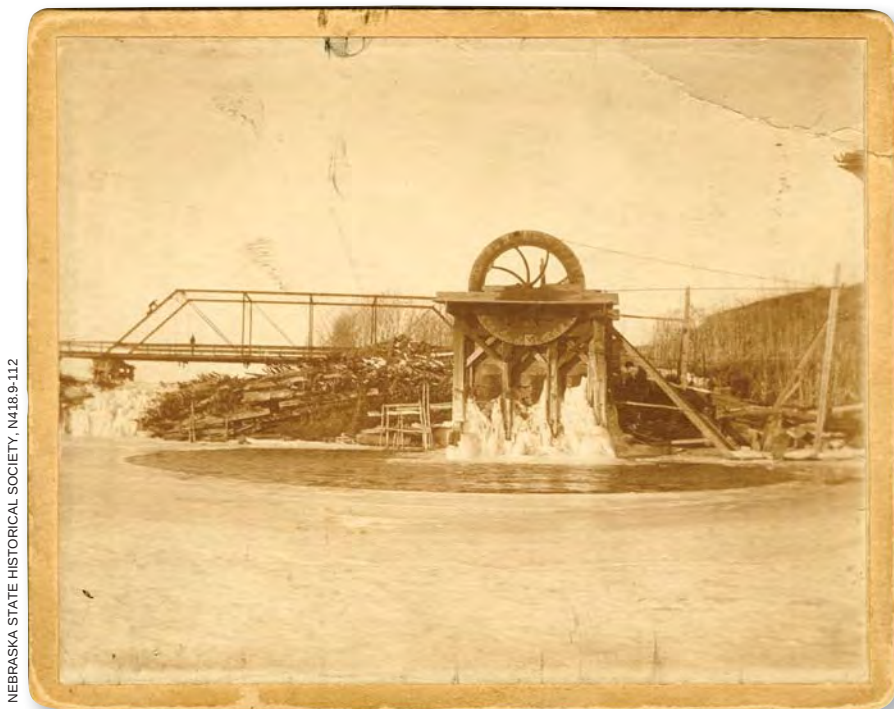
This early view shows the mill penstock with its 10-foot fly wheel that turned a 1-inch wire cable drive to power mill machinery.
