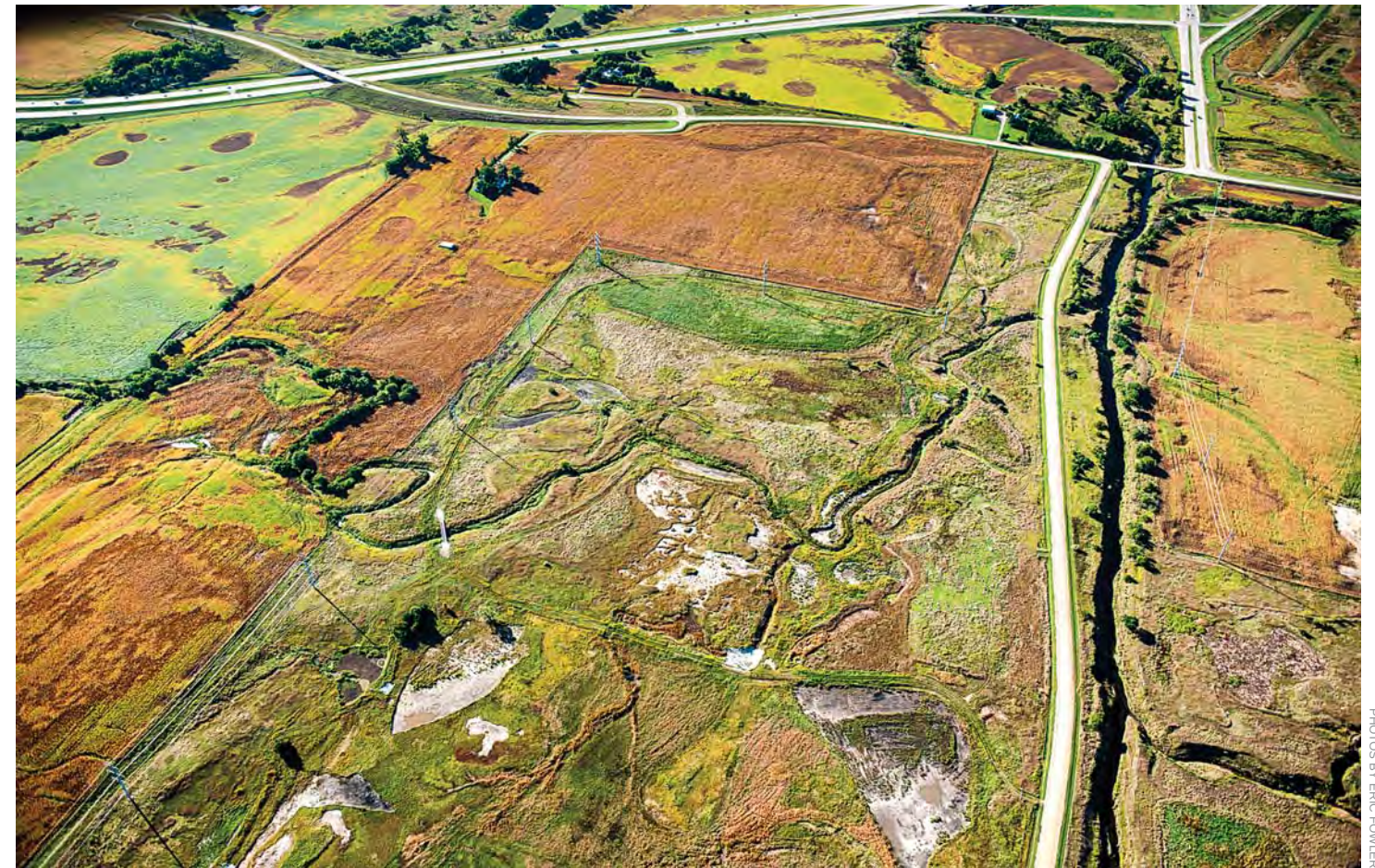
An aerial photo of the Arbor Lake Complex, owned by the city of Lincoln, looking south along North 27th Street toward Interstate 80 on the edge of Lincoln, shows the work that has been done to restore saline wetlands to benefit the Salt Creek tiger beetle and other wildlife. It also shows a channelized stretch of Little Salt Creek, at right, that is home to the insect but once held many more.
