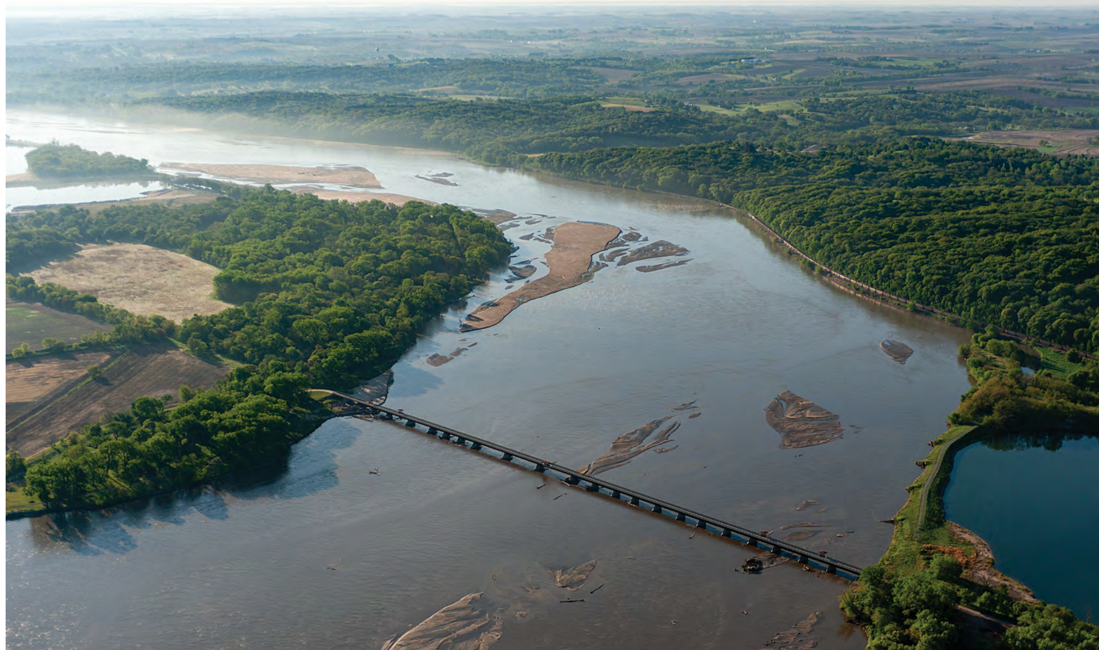
Lied Platte River Bridge is part of the MoPac Trail in Cass and Sarpy counties. It will be part of a yet-to-be-completed hike-bike trail connecting Lincoln and Omaha.
