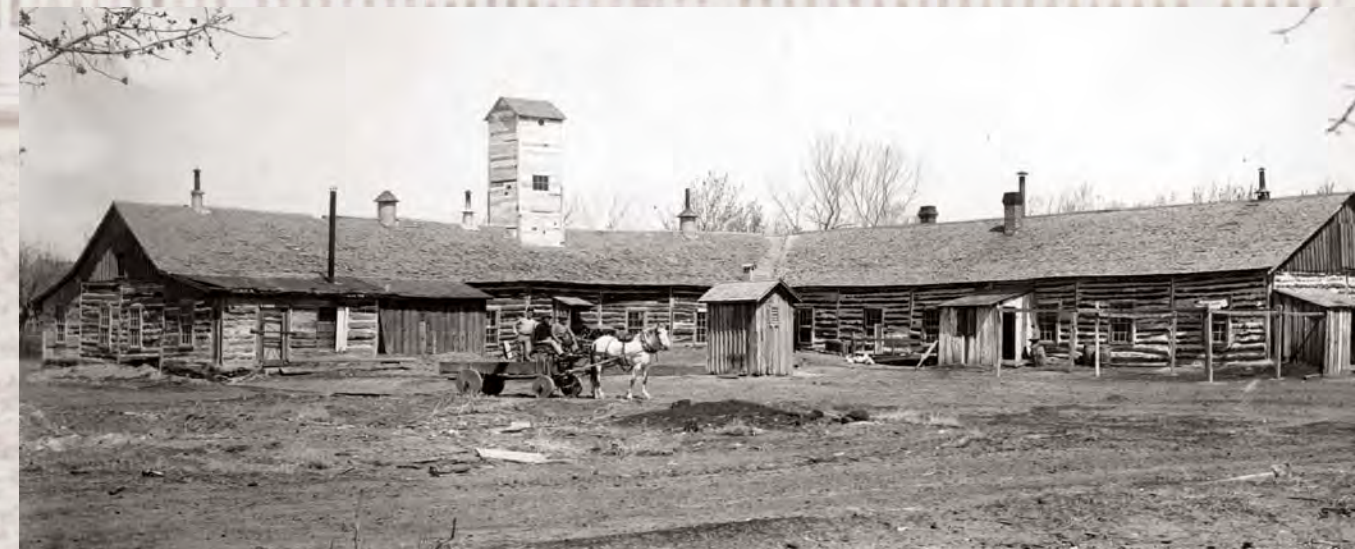
1883 log barracks at Fort Robinson, Nebraska. Founded as Camp Robinson in 1874, the fort served the army until 1948.
