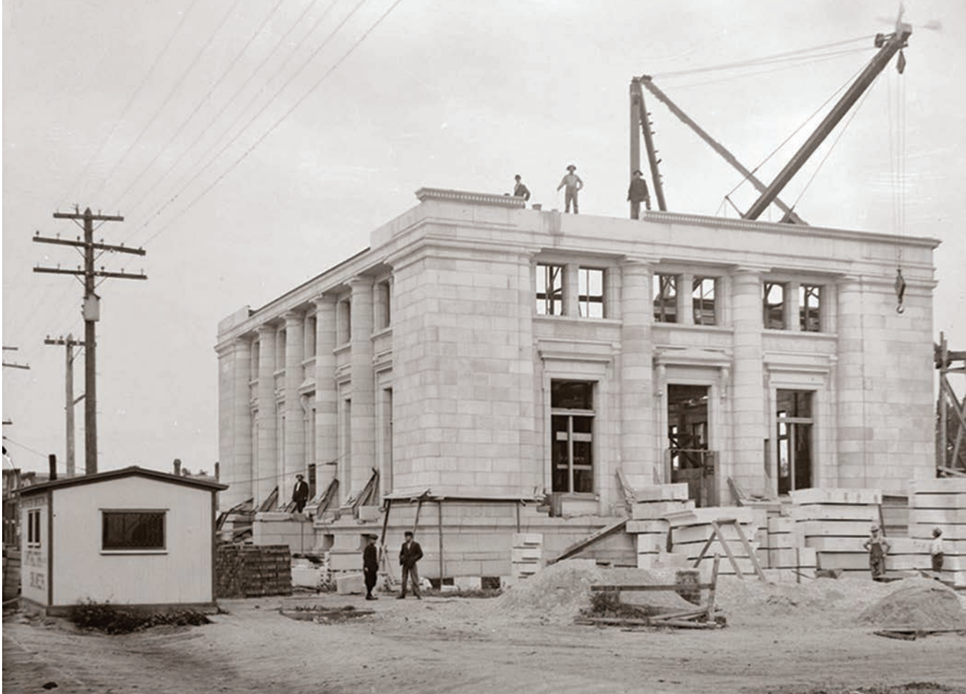
Kearney Post Office under construction in 1907. Today the building is home to the Museum of Nebraska Art and is listed on the National Register of Historic Places. Photo by Solomon D. Butcher. NSHS RG2608-0-2455
