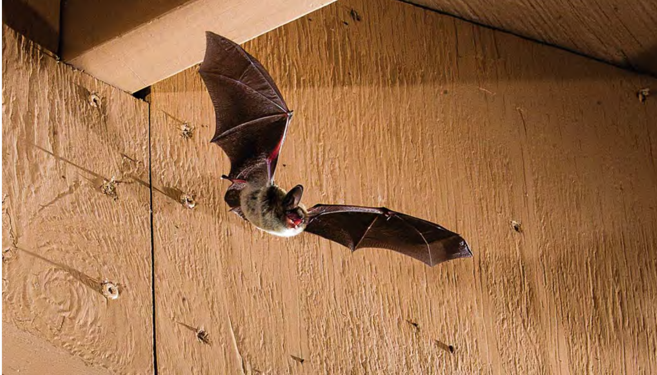
A northern long-eared bat takes flight after emerging from a gap in a cabin wall at Catron Camp and Retreat Center, a Girl Scout camp near Nebraska City. This bat and others established a maternity colony, the first documented in Nebraska, in the space between the walls of several of the cabins and came and went through a 1 centimeter wide opening. They continue to use the site.
