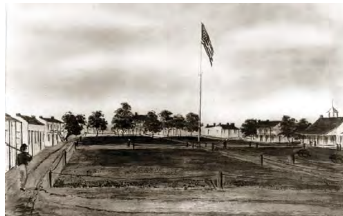
Fort Kearny as it appeared in 1864. NSHS RG2012-4-9.
