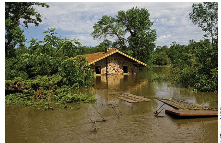
At the crest of the Elkhorn River flood on June 18, water four feet deep lapped at the base of the windowsills of the shelter at Dead Timber State Recreation Area near Scribner. Built by federal work crews during the Great Depression, the shelter sits on an oxbow lake one-half mile from the river.
