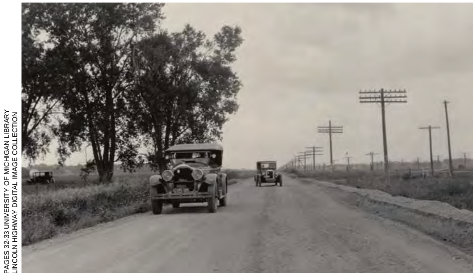
This photo, taken in 1926 between Kearney and Gibbon, shows the method used for graveled the Lincoln Highway - piling the gravel along the side and drawing in one to two inches at a time.
