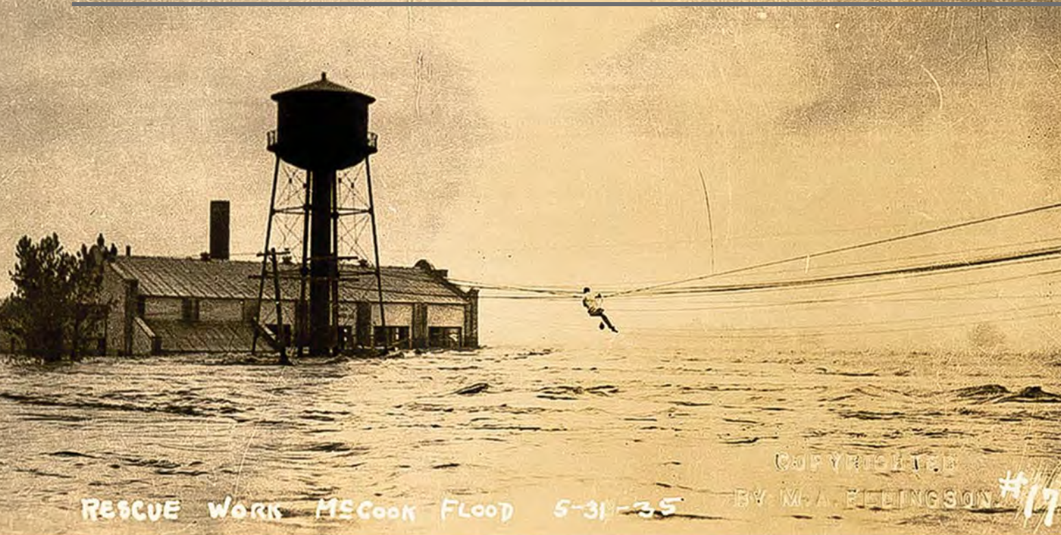
Employee Paul Wilson pulls himself hand over hand to the power plant, bringing a hand line for a telephone cable car to rescue the men.
