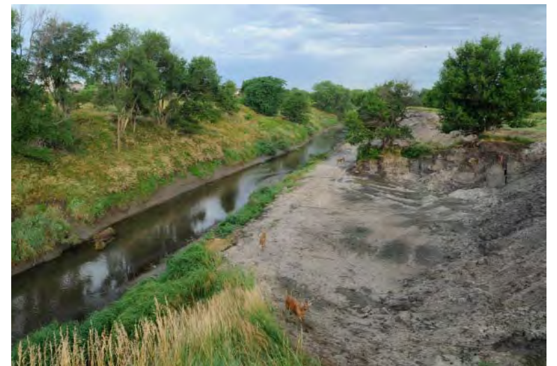
Along Little Salt Creek, excavating and re-shaping a bank to access saline soils and allow for water inundation is the first step in the process.
