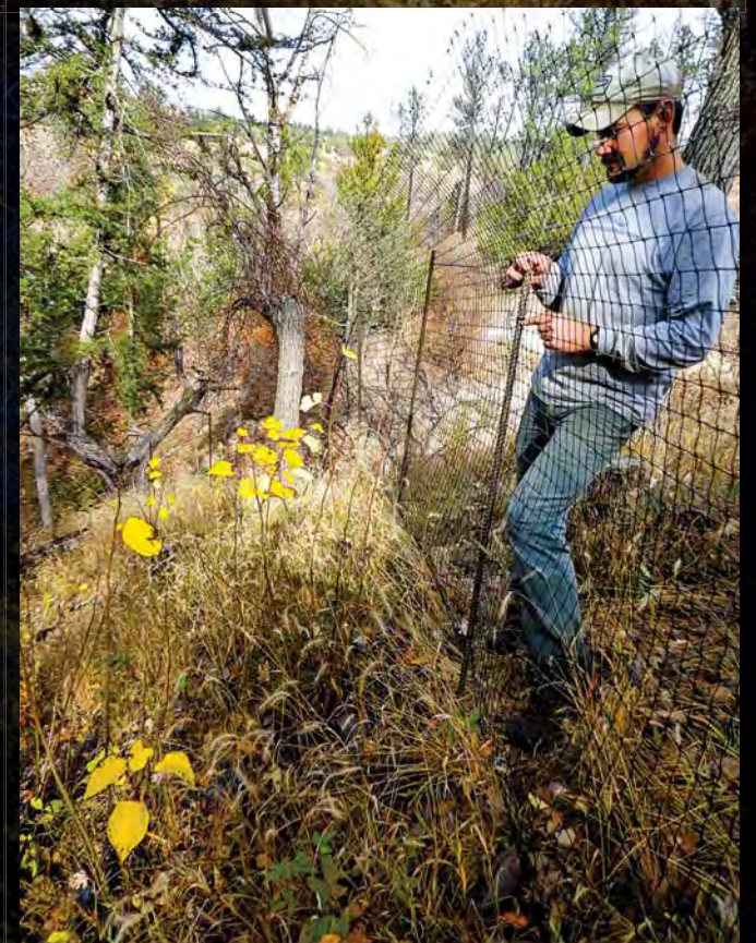
Commission employee Guy McLaughlin installs a fence to protect aspen suckers from browsing deer at Smith Falls State Park.
