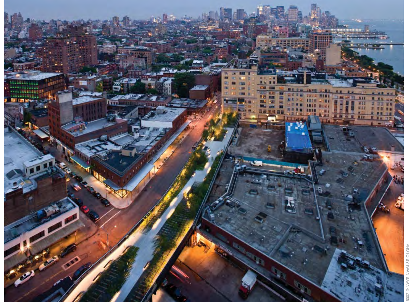
An aerial view from Gansevoort Street to West 13th Street, looking south of the High Line.
