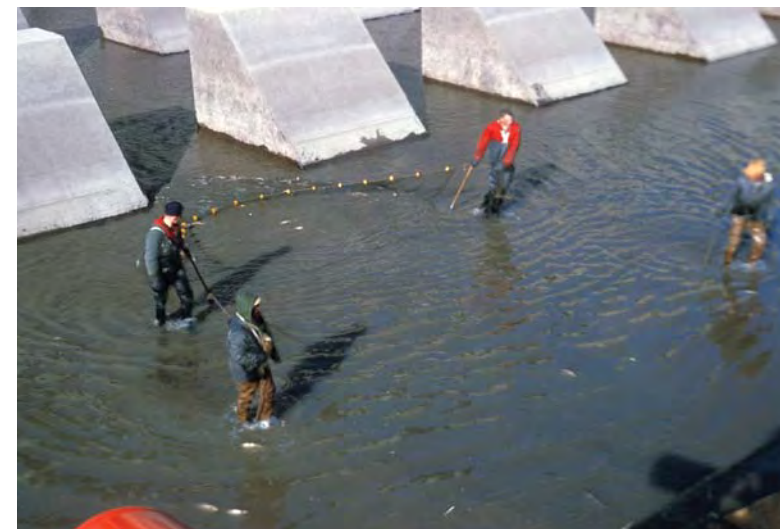
Periodically the settling basin below Harlan County Dam was drained to inspect the structure. The seining crew salvaged the stranded fish to be stocked in the reservoir or elsewhere.
