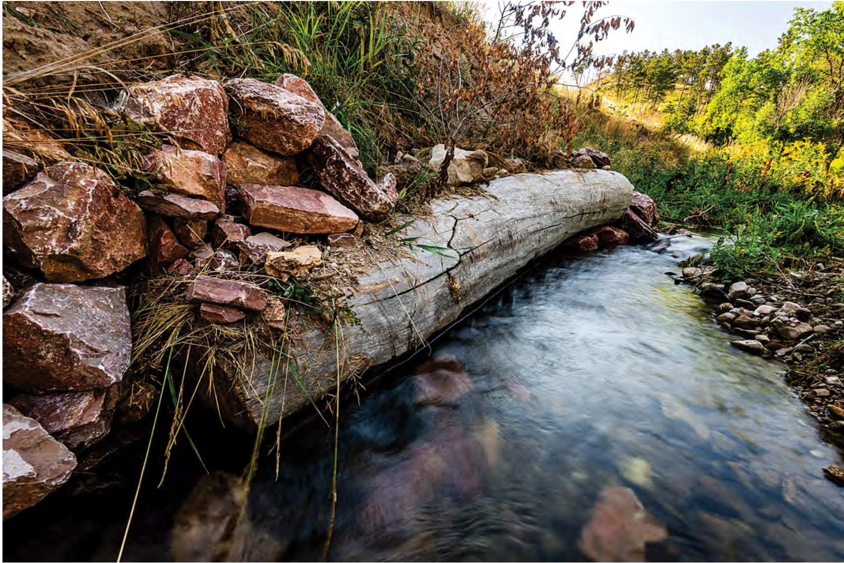
ABOVE: A cottonwood log, harvested from downed timber on site, is among the habitat and erosion control features added to Sowbelly Creek in 2022.
