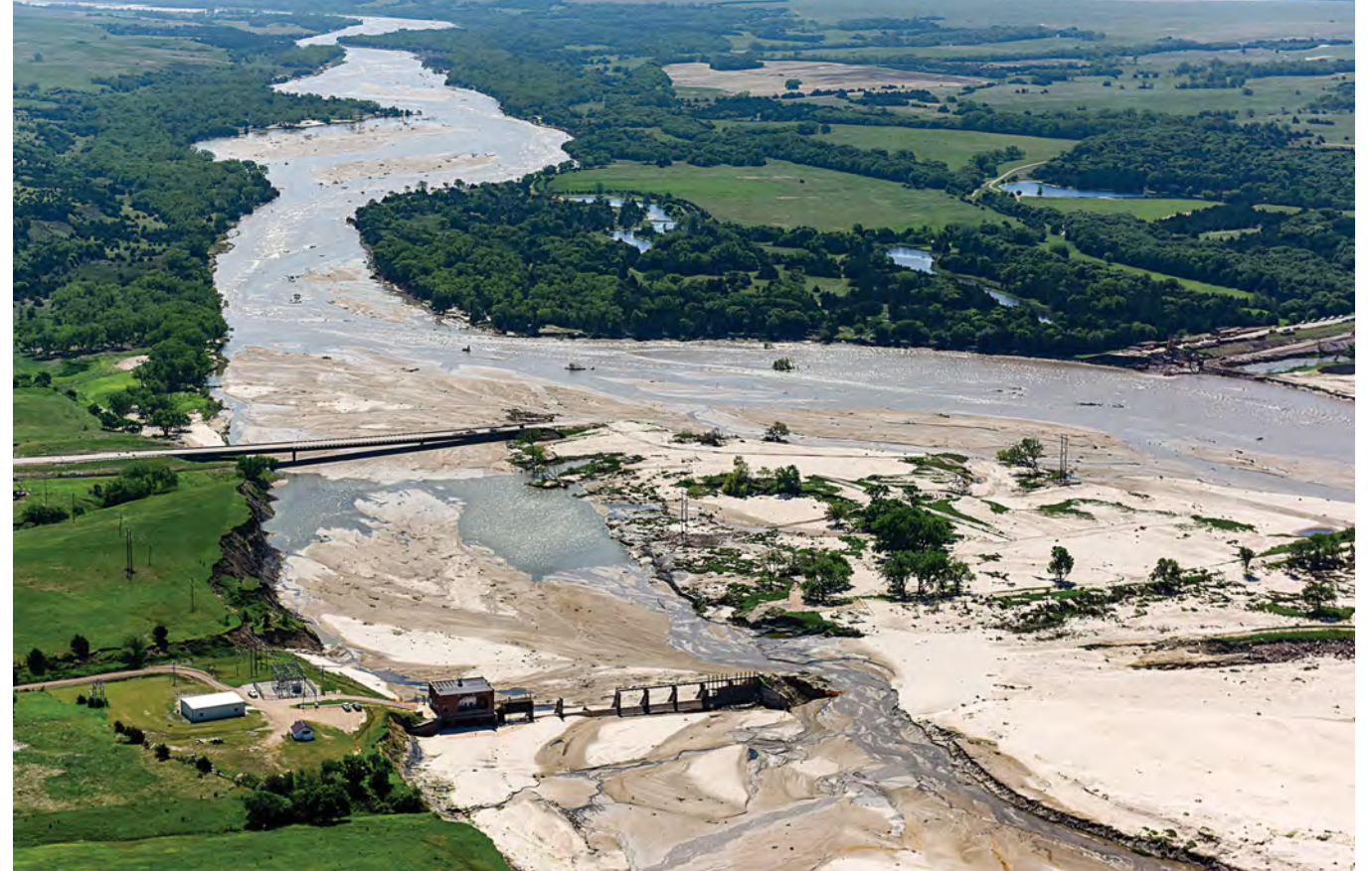
An aerial photo captured in June 2019 looking eastward shows Spencer Dam and the U.S. Highway 281 bridge that were both destroyed by the catastrophic March 2019 flood. With the dam no longer interrupting its flow, the Niobrara River now carries a heavy sand load and has filled many of Allen’s longtime fishing holes along his ranch 5 miles downriver. ERIC FOWLER, NEBRASKALAND
