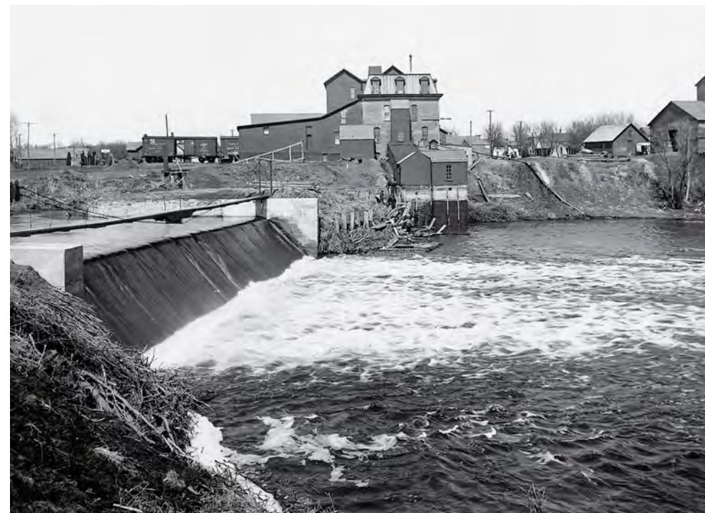
The 1903 dam was stronger and taller to provide more power for the mill.
