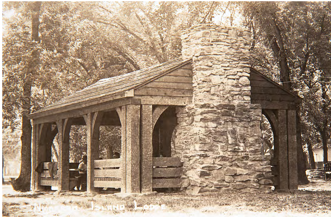
The picnic shelter at Niobrara Island State Park was built with massive, hand-hewn timbers and featured a stone fireplace at one end. COURTESY OF NIOBRARA MUSEUM
