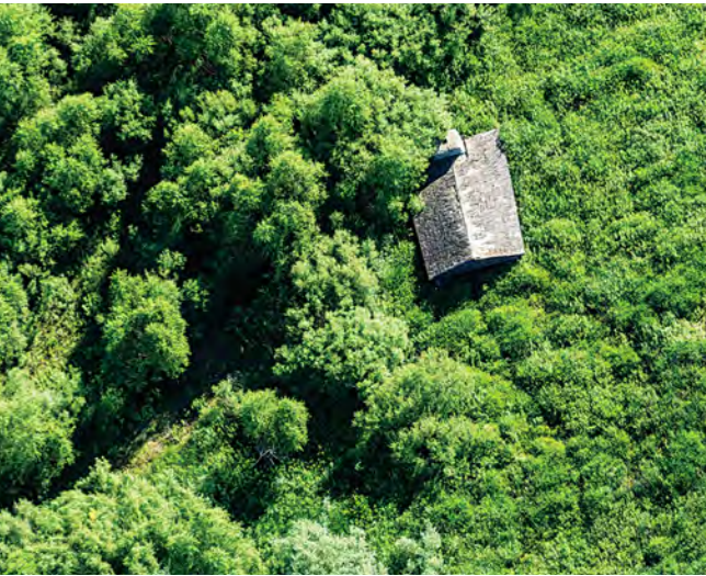
An aerial photo from 2017 shows trees that had grown on the west side of the shelter, roof still intact, obscuring its view from the park. ERIC FOWLER, NEBRASKALAND
