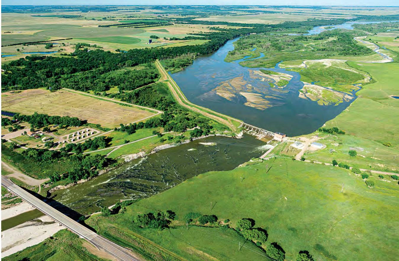
A 2017 aerial photo shows Spencer Dam looking westward. The dam's cement spillway is located on the right while its earthen bank extends to the left. Sand carried downstream by the Niobrara River has settled out of the still water and filled the former lake behind the dam. The clear water flowing out of the dam carried little sand and was highly erosive, scouring deep holes in the river channel downstream. ERIC FOWLER, NEBRASKALAND
