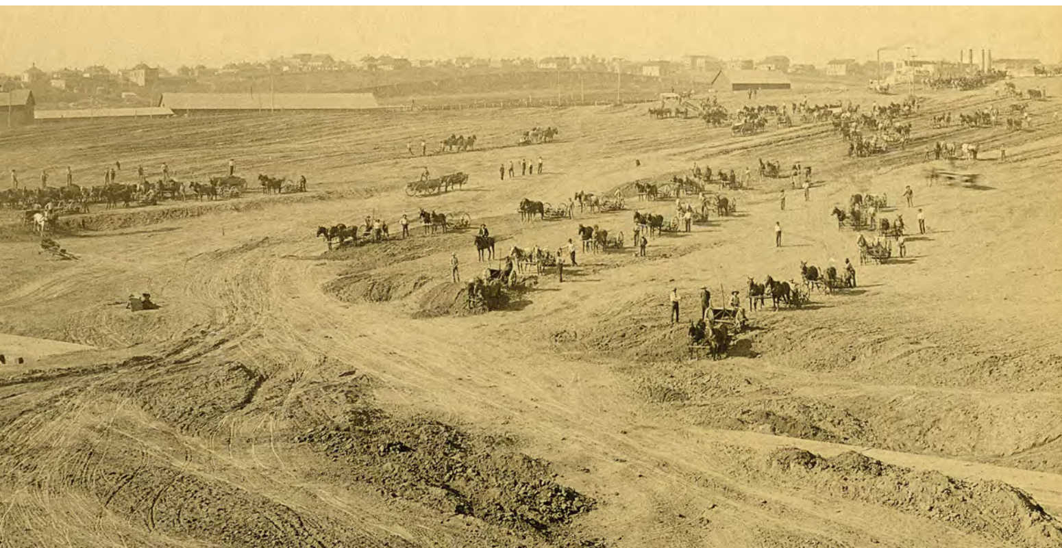
Grading the land ca. 1887. History Nebraska RG1085-77-1
