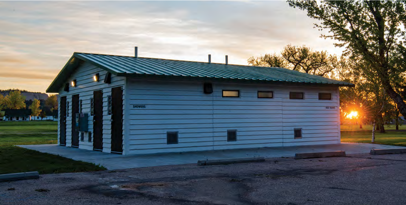
Concrete latrines and showerhouses, such as this one at Fort Robinson State Park’s Soldier Creek campground, are resilient and complement other architecture on the property. JUSTIN HAAG, NEBRASKALAND
