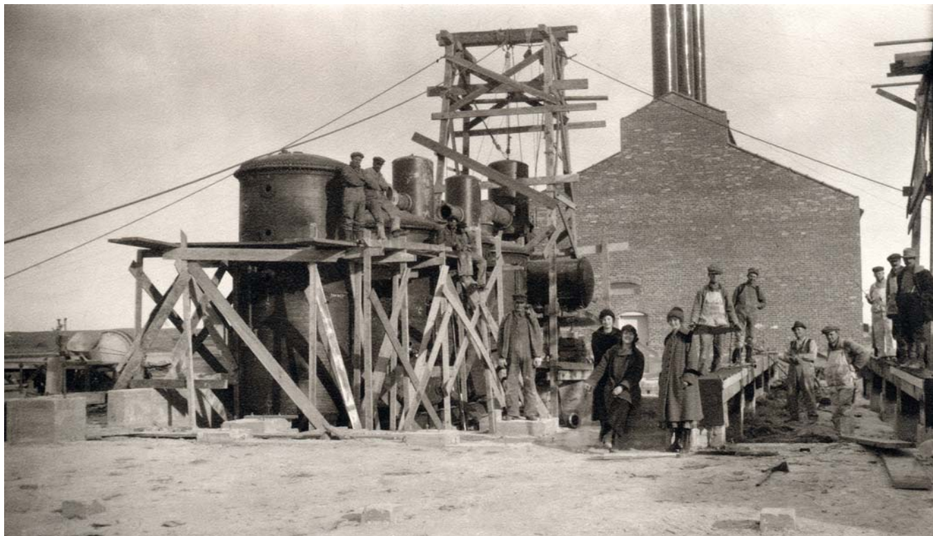
Workers at the Nebraska Potash Company near Antioch posed for a photograph in front of the power plant and next to “evaporating pans” that were being installed. The negative identifies the photographer as Hager, perhaps a student of Barbour.
