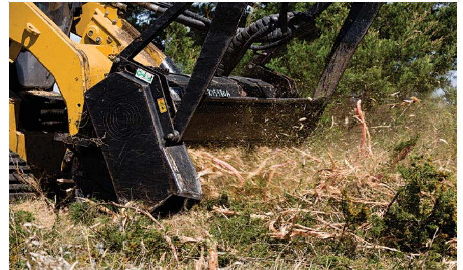
Contractor FDC Enterprises of Ohio used a fleet of skid steers equipped with chipper heads to remove hundreds of acres of invading cedars and planted tree rows. Chipping cedars is often more efficient than shearing, piling and burning.
