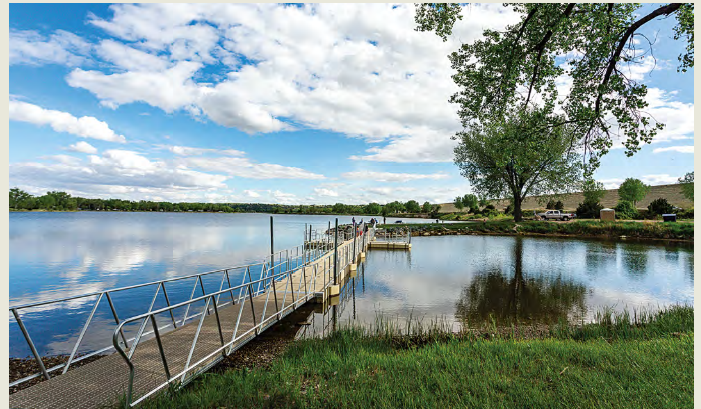
A 160-foot floating bridge connects a peninsula to the northwest shore of Lake Ogallala. A portion of the funds for this angler access bridge was provided by the Central Nebraska Public Power and Irrigation District.
