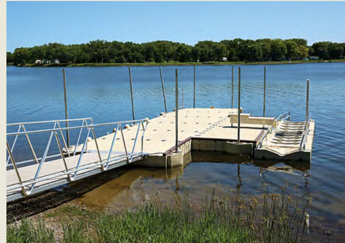
A new boat dock was installed at Lake Ogallala on the west side, which features an accessible kayak and canoe launch, the first of its kind in western Nebraska.
