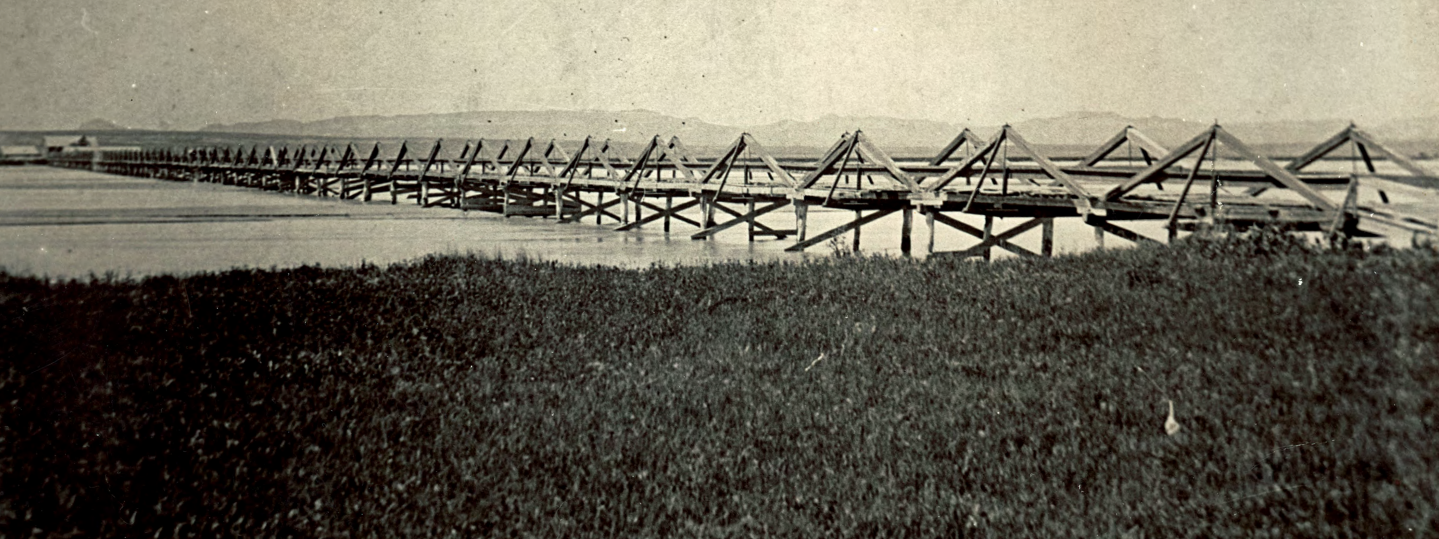
Camp Clarke Bridge near present-day Bridgeport, looking south toward the Wildcat Hills. HISTORY NEBRASKA, RG3289-0-24-A2
