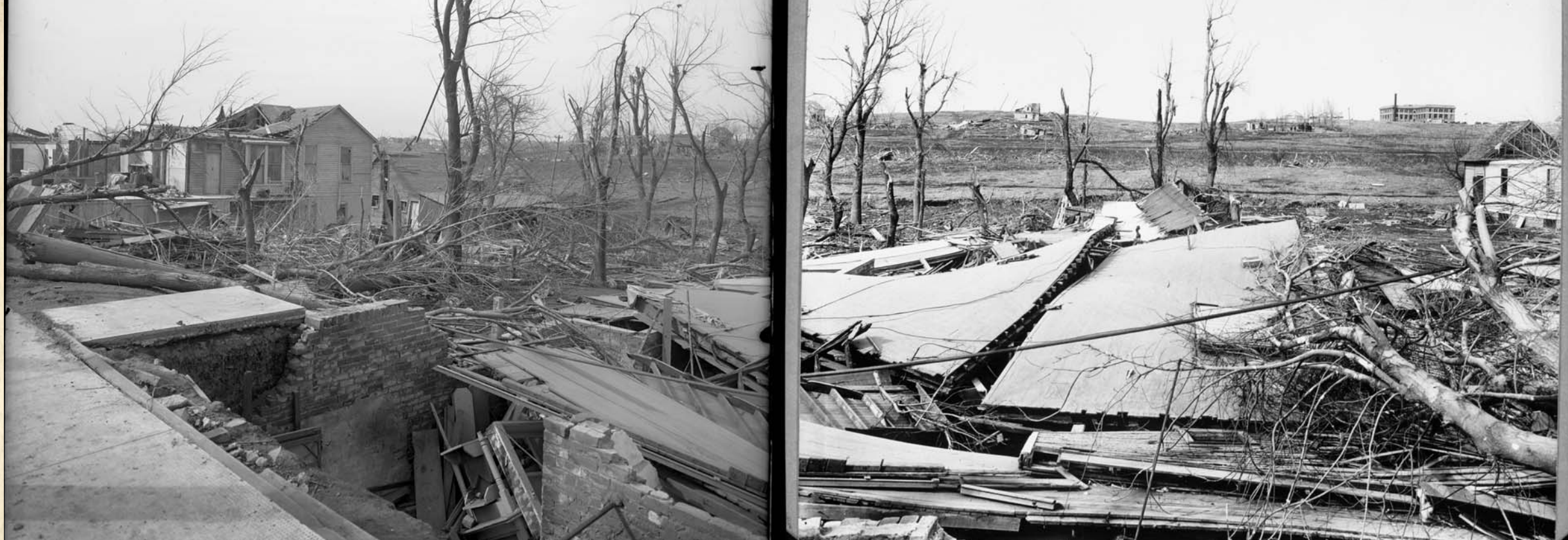
This panoramic photo shows homes on the southwestern edge of Omaha along Leavenworth and 49th streets, including this one blown from its foundation. Twelve people lost their lives in this vicinity. On the hill at right is the University of Nebraska Medical College building.
