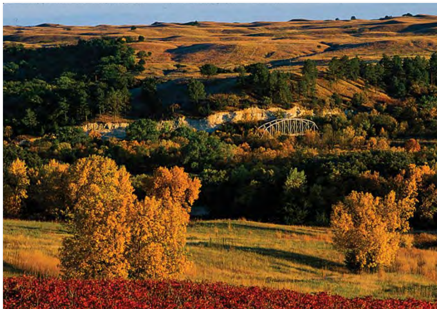
The Norden Bridge spans the Niobrara River on The Nature Conservancy's 56,000-acre Niobrara Valley Preserve located in north-central Nebraska. The Preserve is one of Nebraska's botanical hotspots supporting over 580 plant species.
