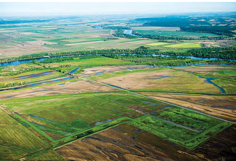
Low berms built on Langdon Bend Wildlife Management Area near Nemaha hold back natural precipitation as well as pumped well water to create wetland habitat that is lacking on the floodplain along the channelized portion of the Missouri River.
