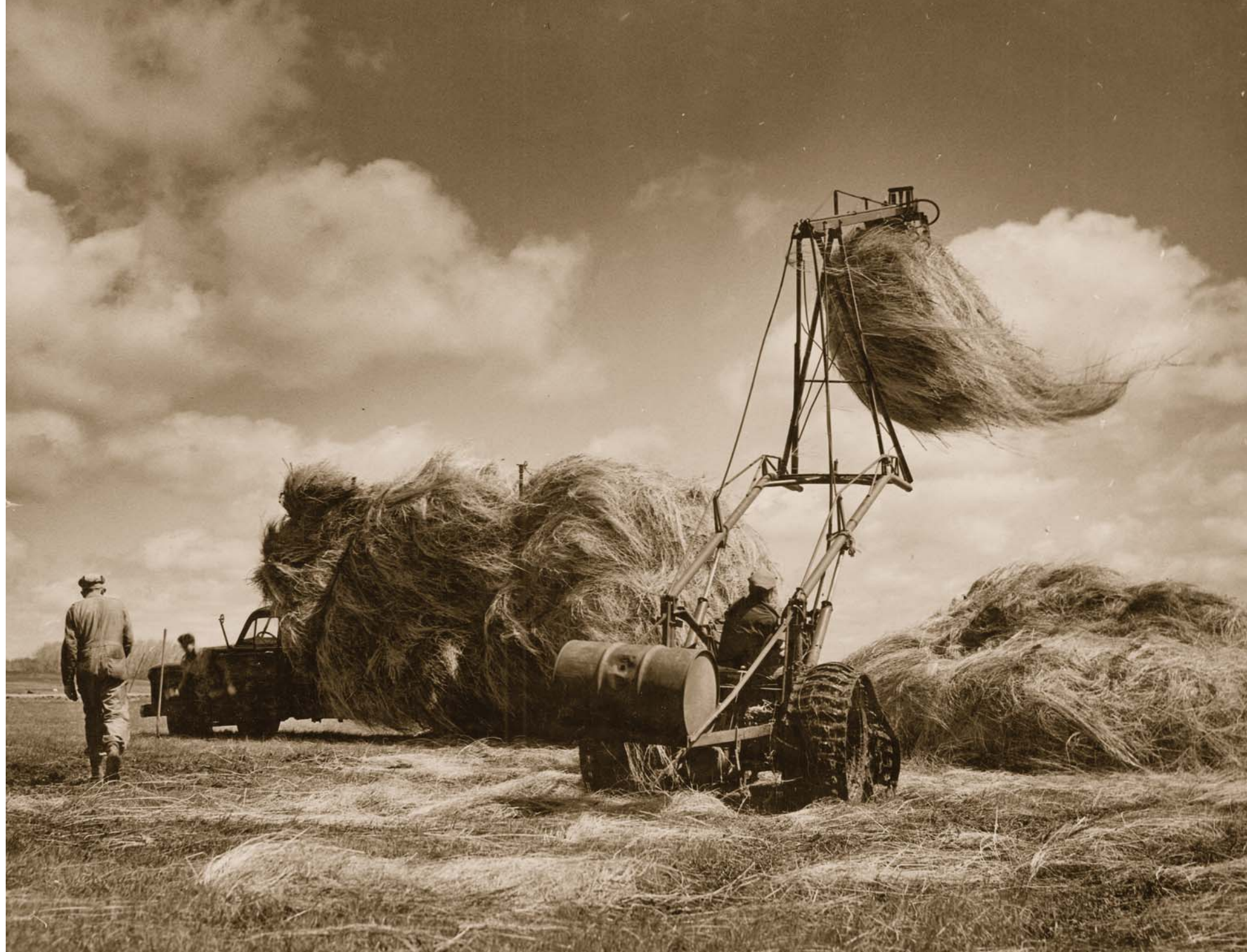
Saunders invented or modified equipment to harvest prairie cordgrass from wetlands near Columbus for the manufacture of target mats.
