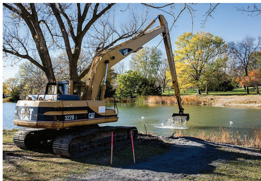
Several lakes at Windmill State Recreation Area were excavated to provide depth to ensure shallow areas remain connected during low water. ERIC FOWLER, NEBRASKALAND
