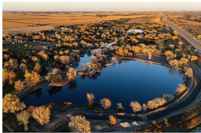
A channel cut around Lake No. 1 at Windmill State Recreation Area will carry floodwaters away from the area. ERIC FOWLER, NEBRASKALAND
