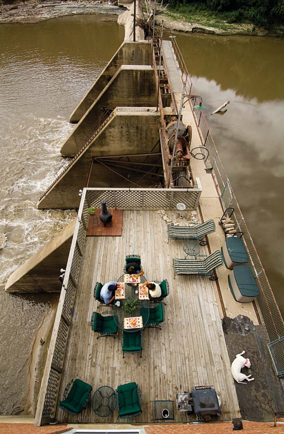
A deck above the first gate on the dam, which was sealed with concrete after it fell into disrepair, provides the Petersens a place to relax.
