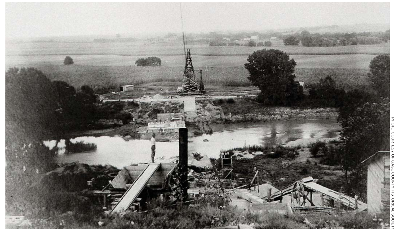
Work on the Barneston Dam began with the base of the powerhouse on the east bank of the Big Blue River in 1919. Rock was quarried from the west bank for the concrete, which was mixed and hauled across the river on a cable strung between two derricks.
